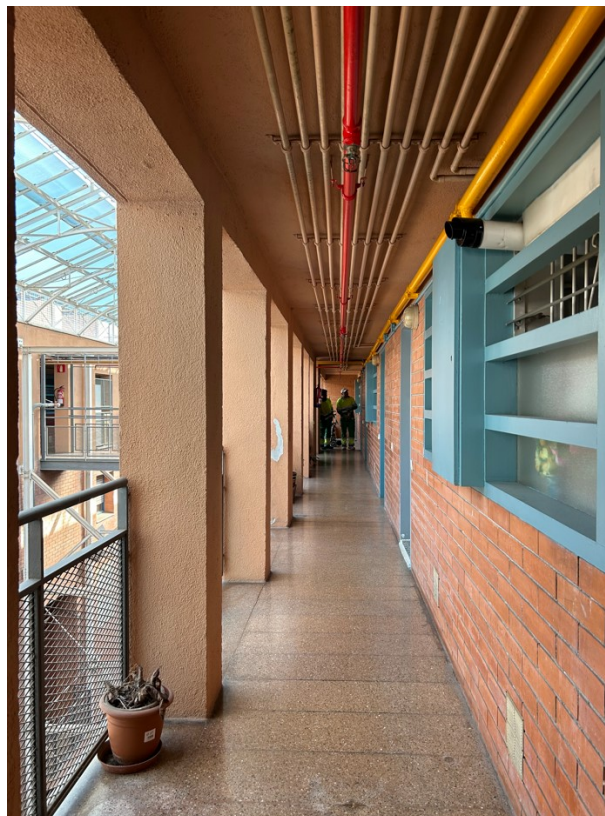
F2 – Façana a pati interior
