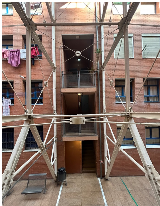
F2 – Façana a pati interior
